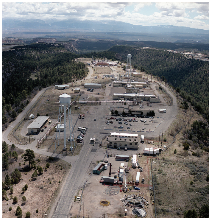
Technical Area 21 during decommissioning and decontamination.
