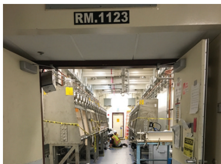
Contractors installing glovebox trains at RLUOB.
